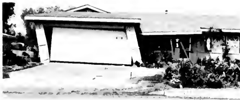
Photo 1. Example of damage incurred by residential structures in zone of ground rupture and intense shaking. Failure of garage was primarily a result of horizontal motion. Photo courtesy of City of Los Angeles Department of Building and Safety.
